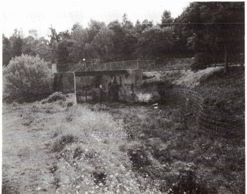
Natural Bluestone Wall & Mill Race Below
